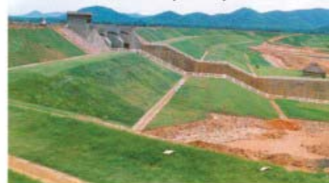
Kovvada Kalava Spillway
